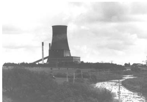
Figure 1.4 Power Station, Bellacorick, County Mayo, Ireland. The power station is fed by local peat bogs
